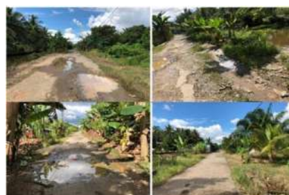
Fig.3. Country road conditions
