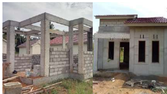
Figure 8. Wall and Roof Works
